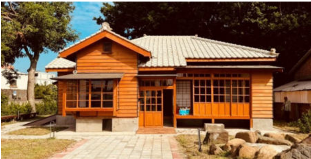
▲ Figure 2-21 Results of the restoration of the historic building “former police dormitories” in Lunbei Township, Yunlin County
