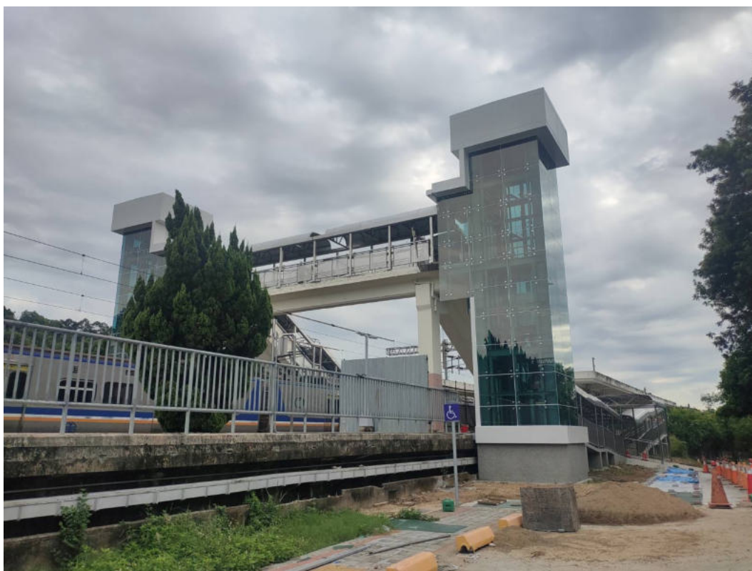
▲ Figure 2-18 Installation of an accessible elevator at Taiwan Railway's Zaoqiao Station
